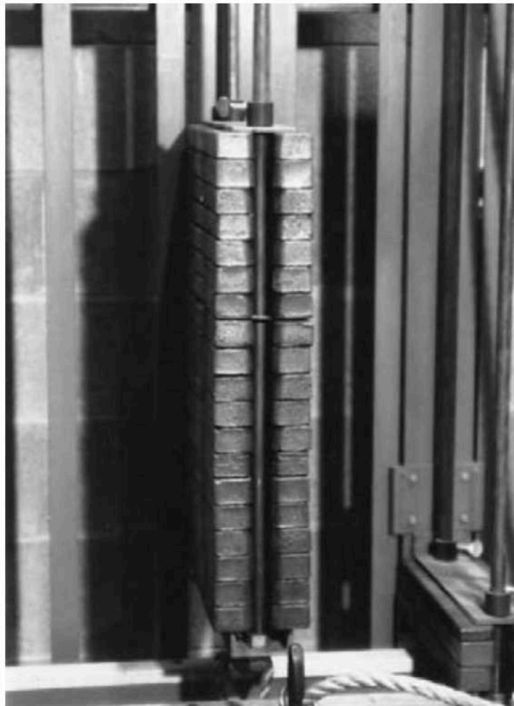
Fig. 4.22. Counterweights with spreader and lock plates in place
