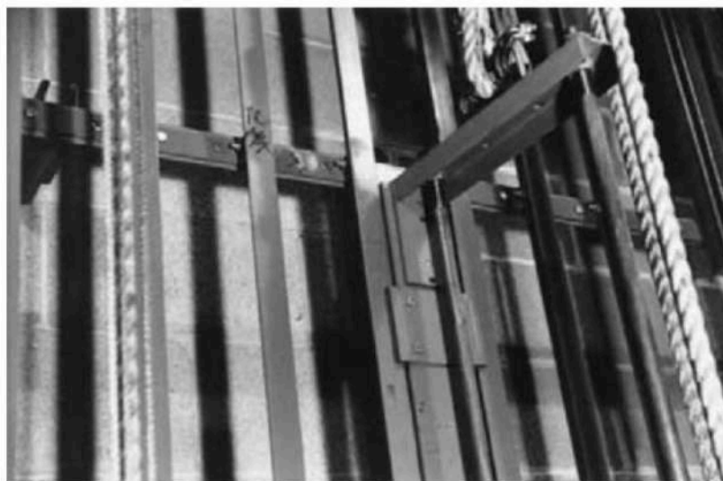
Fig. 4.25. T-bar-guide counterweight set
