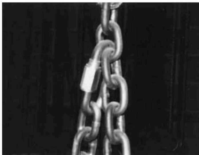
Fig. 4.10. Loose Quick Link on trim chain
