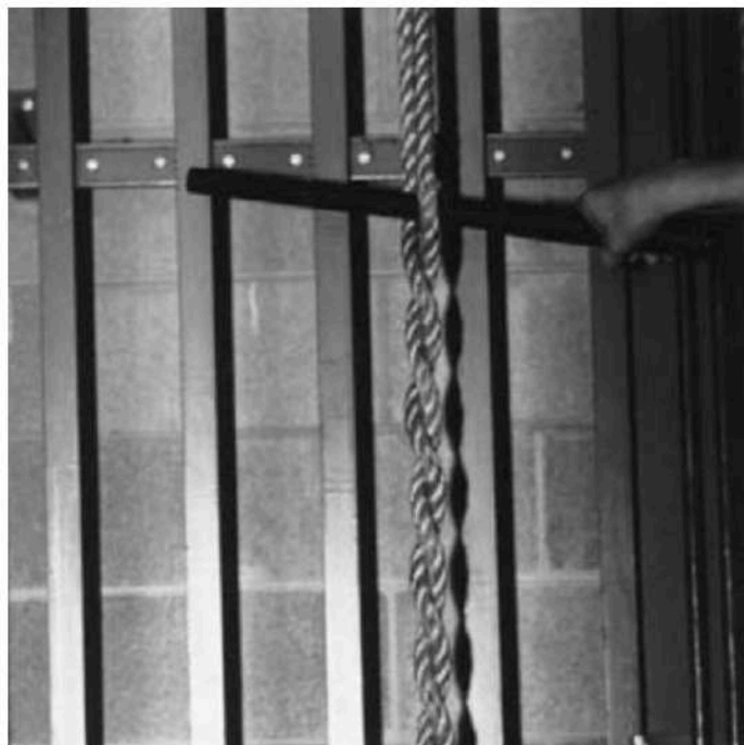
Fig. 4.32. Belaying pin in hand line
