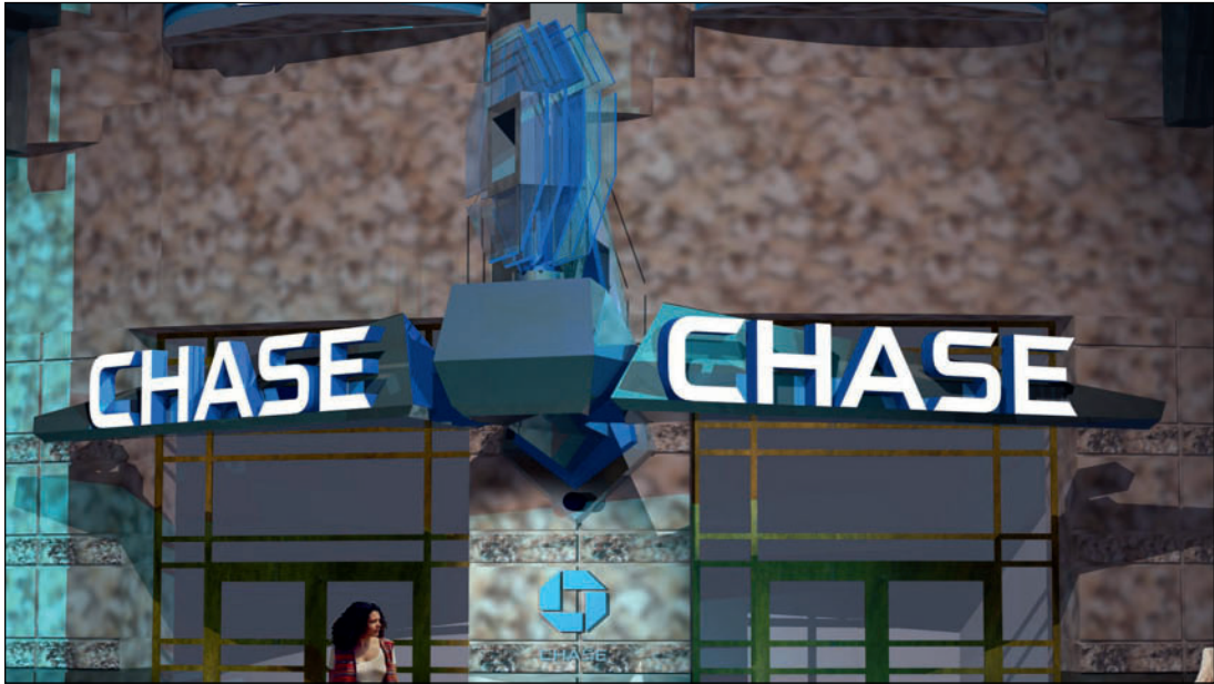
Chase Bank Flagship Signage at 3 Times Square Rendering and animation by the author.
