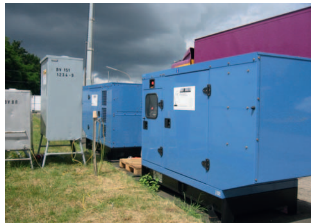
FIGURE 12.11 Transformer. (Photograph by Paul Dexter.)
