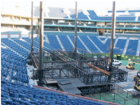
FIGURE 14.20 Four-pole freestanding roof being assembled. (Photograph by Brown United.)
