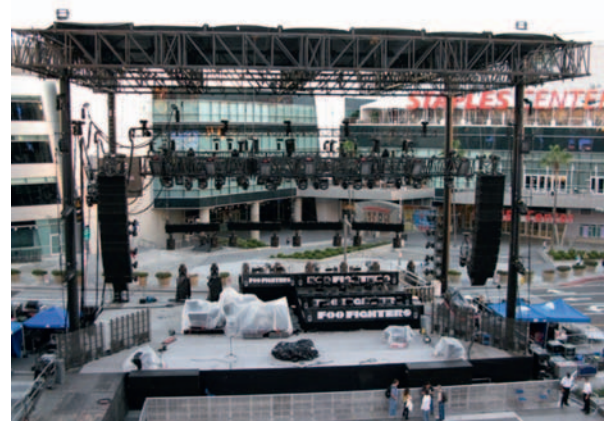
FIGURE 14.21 Four-pole roof raised with speaker clusters and lighting trusses supported. (Photograph by Brown United.)
