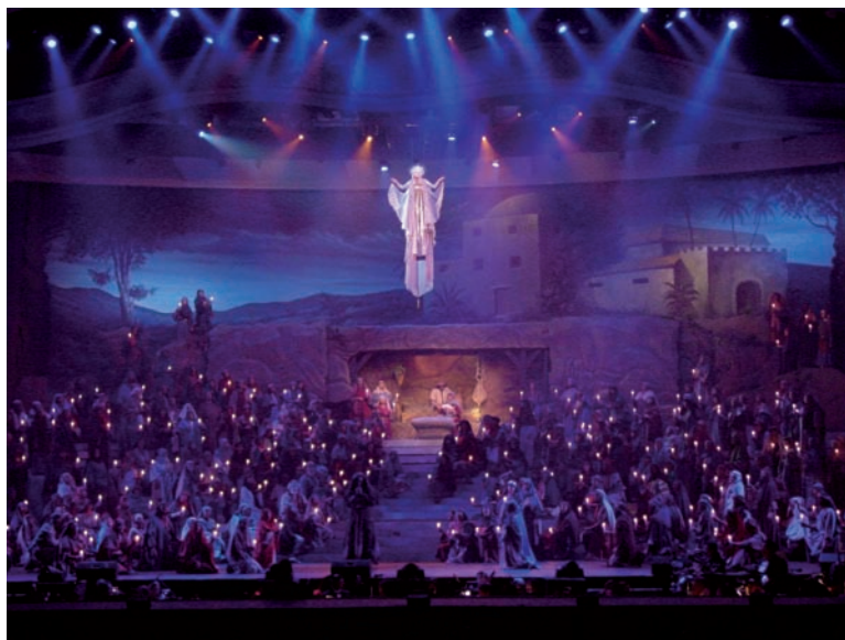
Figure 25-6 Prestonwood Baptist Church in Plano, Texas. Automated lighting is gaining popularity in the modern house of worship. It is used for a variety of functions, including key lighting, special effects lighting, color wash, and architectural lighting. (Photograph courtesy of Brawner and Associates. Lighting design by Donnie Brawner.)
